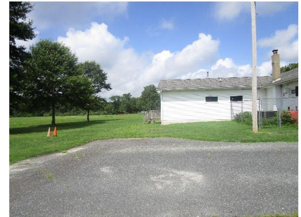
A rain garden can be installed at the southeast corner of the building to capture, treat, and infiltrate stormwater runoff from the rooftop. A preliminary soil assessment suggests that more soil testing would be required before determining the soil's suitability for green infrastructure.
