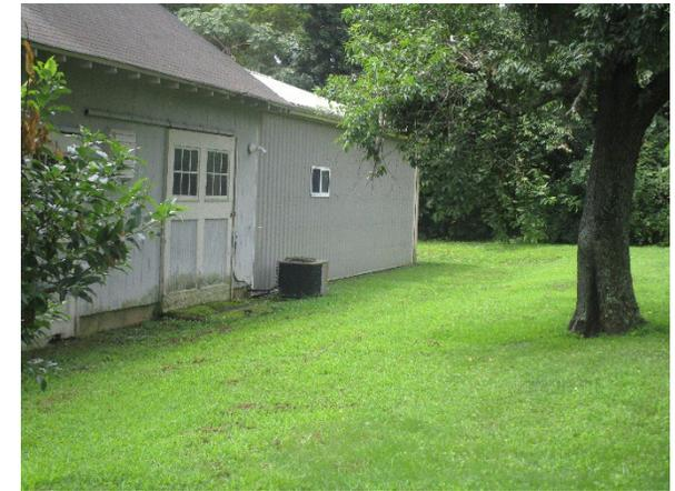
A rain garden can be installed in the turfgrass area on the north side of the building to capture, treat, and infiltrate stormwater runoff from the roof. A preliminary soil assessment suggests that the soils have suitable drainage characteristics for green infrastructure.
