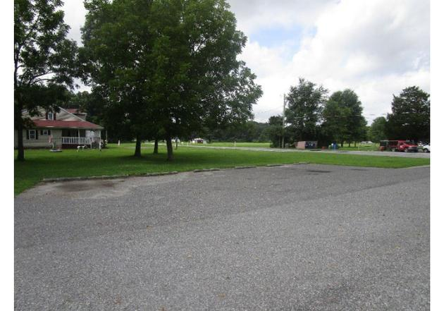
Pervious pavement can be installed in parking spaces to capture and infiltrate runoff from the parking lot and the rooftop from a downspout at the southwest corner of the building that can be disconnected to flow onto the parking lot. A rain garden can be installed on the north side of the building to capture, treat, and infiltrate rooftop runoff. A preliminary soil assessment suggests that more soil testing would be required before determining the soil's suitability for green infrastructure.
